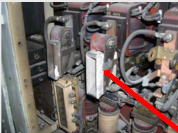
Switch gear flash guard and electrical wiring
